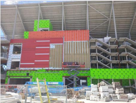
The first phase of a \$120 million 2-year renovation project is underway and WrapShield SA Self-Adhered WRB/Air Barrier membrane is protecting the new 30,000 seat stadium. WrapShield SA was installed over the last several months, even in below freezing temperatures and wet weather. Deputy Mayor Kelly notes, "The improved stadium will become an incredible sport destination that will be enjoyed by fans from across Toronto and beyond."
