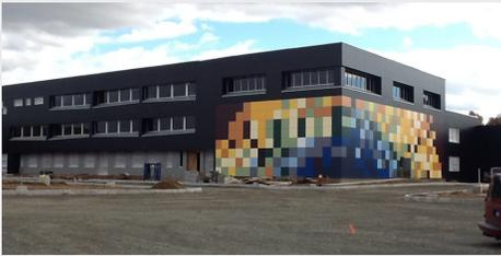
Behind the colorful cladding, over 60,000 sq.ft. of WrapShield SA Self-Adhered WRB/Air Barrier is protecting the state-of-the-art CREC Academy of Aerospace and Engineering in Windsor, CT.
